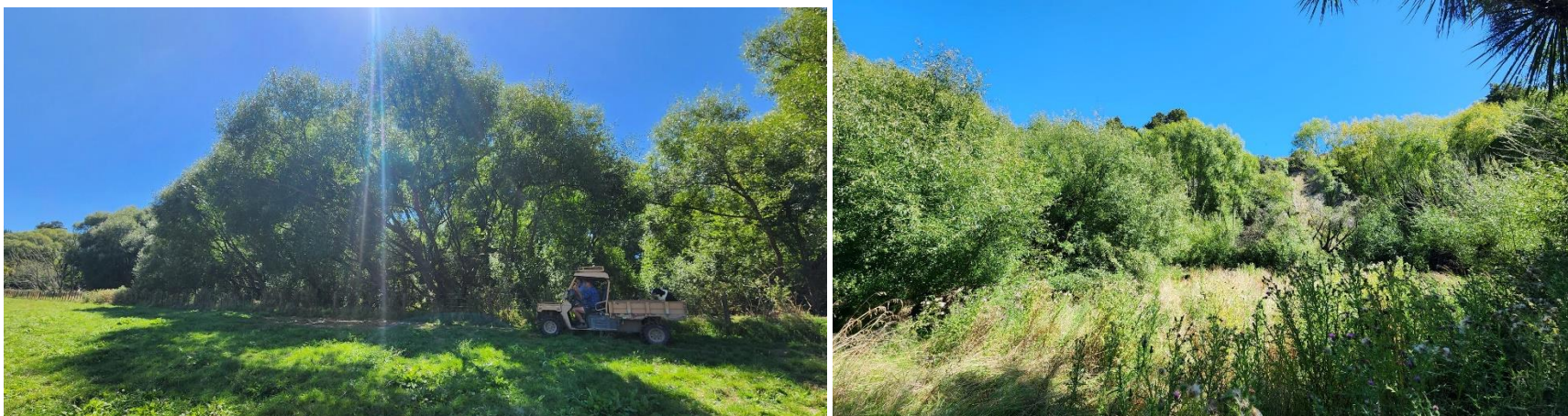
Figure 7 - Large willows remain on several portions of the main channel. It would be beneficial to remove these and keep these areas willow free through maintenance.
