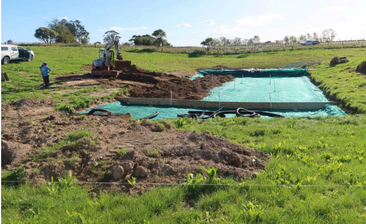
Figure 6 – Existing denitrification bioreactor in the sub-catchment.
